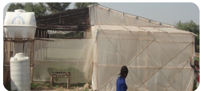
Greenhouse constructed by steel (left); constructed by wood (right)
