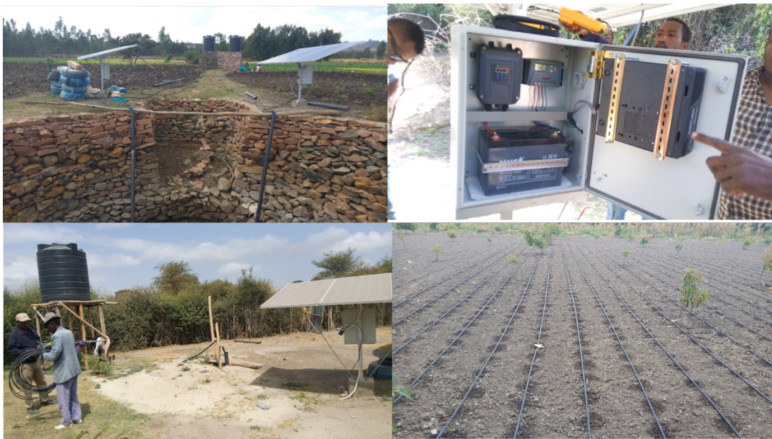
Figure 11: Solar pumped drip irrigation system
